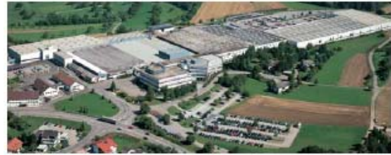
Main factory of the Homag Group in Schopfloch, Baden-Württemberg, Germany.
